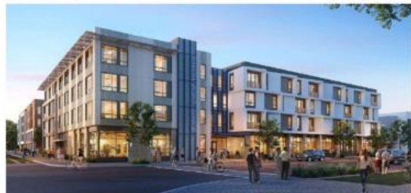
Eden Housing and Alameda Point Partners are constructing the 60-unit Alameda Point Senior Apartments at Alameda Point, a creative reuse project just south of Oakland, Calif.
