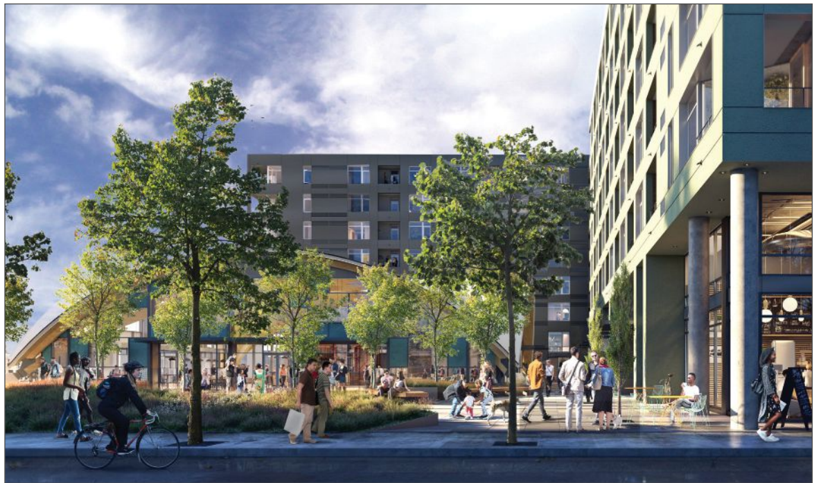
Mithun’s Splash Apartments in Portland, Ore., include a plaza area with custom-designed benches and a water feature that is available to residents as well as to the public.
