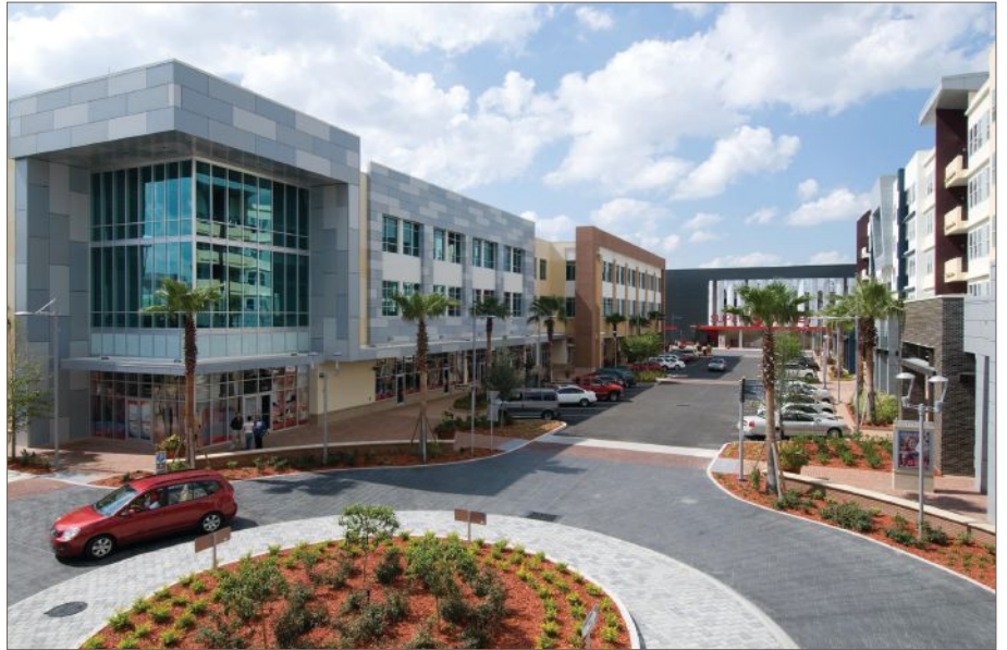
SoDo (south of downtown) in Orlando, Florida, is a 22-acre, transit-adjacent urban infill mixed-use project. It features retailers like TJ Maxx and a Super Target with rooftop parking. It was designed by CUPKOVIC architecture.
