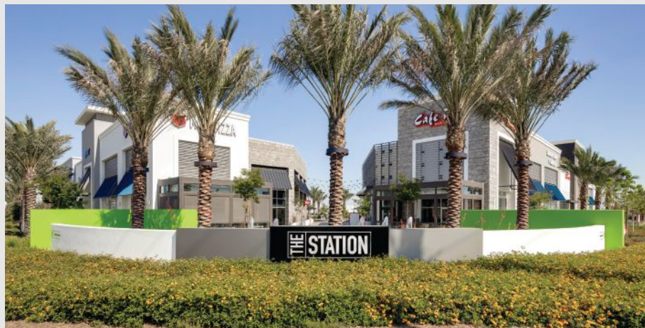
The Station is the 60-acre retail component of Goodman Commerce Center. It will include a 650,000-square-foot power center. (Credit Goodman Birtcher)
